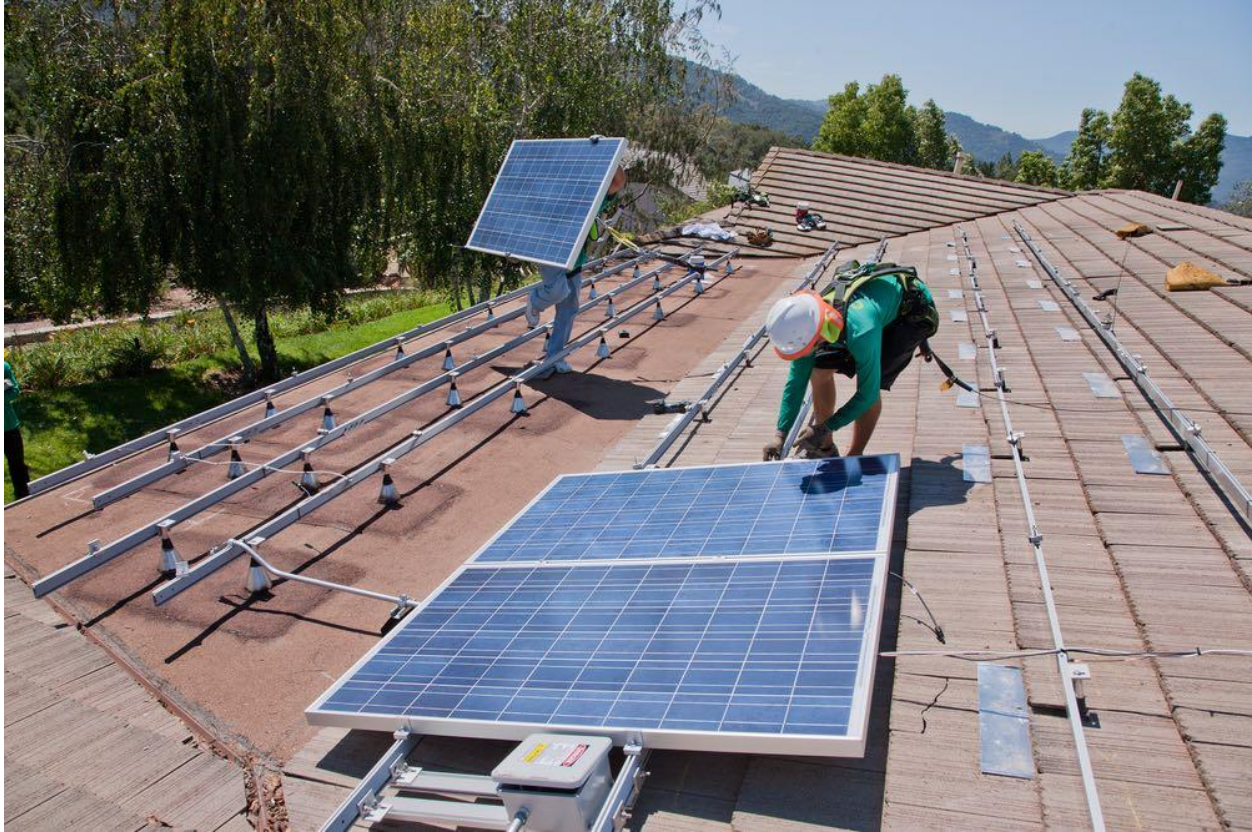
Figure 3.4: General structure of PV System being installed in a roof.
